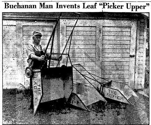
BUCHANAN, Mich., Sept. 13.-A leaf rake has been invented by William Nelson, 65, of Buchanan for which he has the patent pending. The rake is a metal box 38x36x 12 inches which slopes downward toward a row of metal teeth, which form the rake, as shown here. The vehicle is pushed around the yard, and the momentum pushes the leaves upward into the box. (Smith Photo.)
