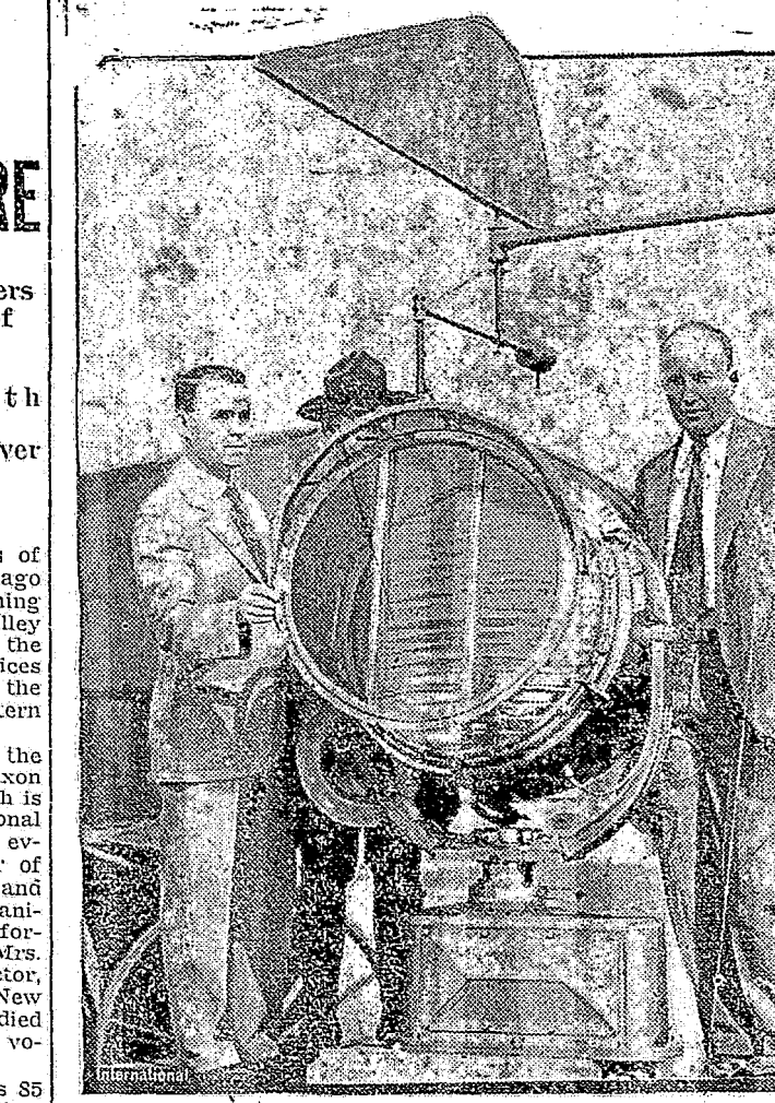
Maj. Francis Boyle, Capt. J. H. Palmer and Capt. Dudley Howard, left to right, inspecting the new windage beacon undergoing tests at Rolling Field. This revolving beacon with the wind direction indicator was invented by Major Boyle and is so designed as to throw a colored beam down wind for a distance of from one to two miles as an aid to pilots making landings at night.
