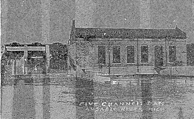
FIVE CHANNELS DAM ON AU SABLE RIVER
