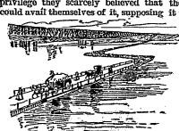
PONTOON BRIDGE AT NEBRASKA CITY. be impracticable. However, the bridge has been built, and it is said to be the largest pontoon bridge in the world. The especial feature is a V shaped draw, with the angle of the V down stream, which the current may open whenever required. The draw is so constructed as to be closed by one man. From the Missouri to the Oxus is a big step. The Central Asian railway has been
