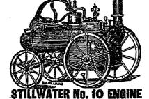
For wood or coal fuel; has a return flue botter makin it very economical in fuel. Its cylinder is 7×12. We also make the Stillwriter No. 12, and th Minnesota Giant Farm Engines, each ha ing return fues, and fitted for burning straw, wood or coal. All these Engines are made and finishe in the wood perfect maner, and Traction Attach ments can be furnished with any of them if d wired. If For Price Lit and Curculars, addres
