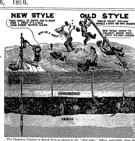
The Chapman Tabular or Bored Well as shown in the "New Style," differs materially from the Position of Screen and Valves in Well.
