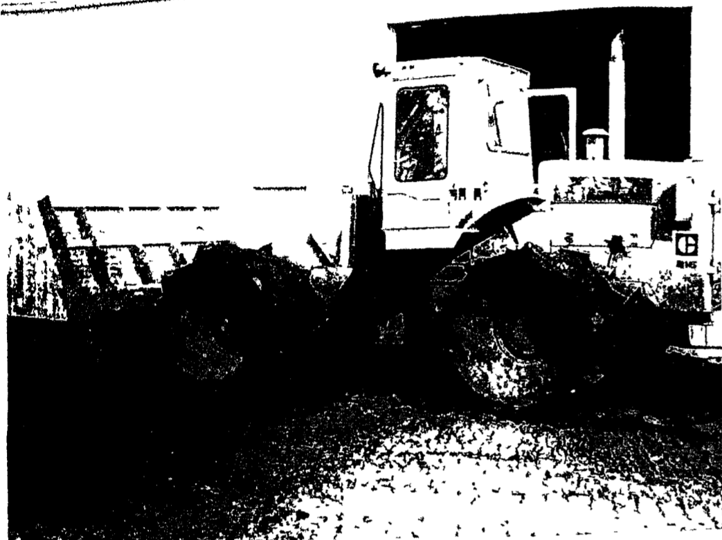
This is the new Caterpillar compactor now owned by the Southeast Berrien County Landfill Authority.
