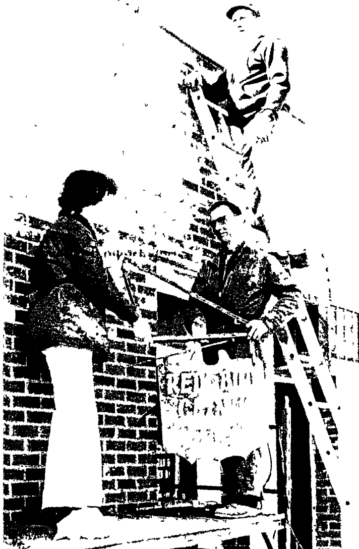
Kris DeSomer, Pete Walls and Arvel Johnson erected the new sign for Red Bud Clinic, which houses the offices of Dr. Jack Barden and Dr. Don Brogan.
