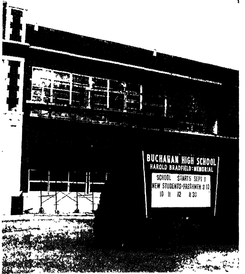
The installation of new windows in Buchanan High School was continuing this week. The work is the first phase in a three-phase energy conservation project for the district. A bond issue to fund the work was approved by voters last year.
