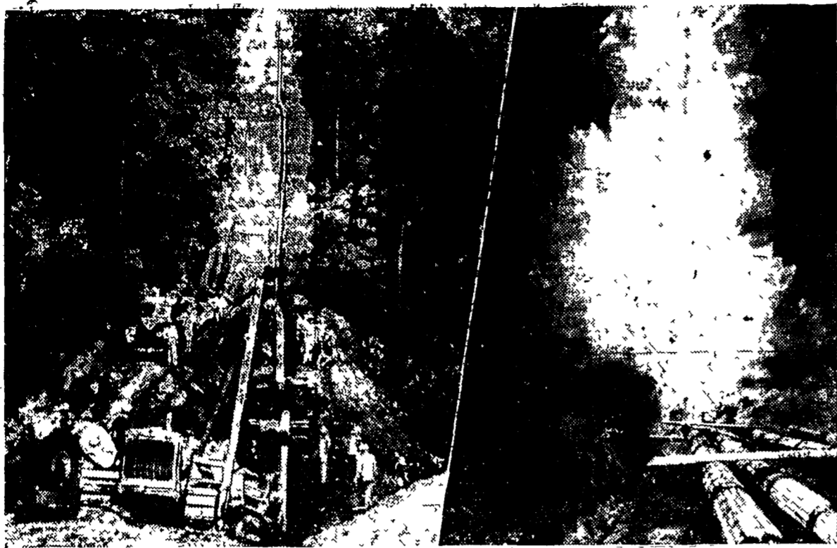
When a petroleum pipe line is being built to supply war industries with the precious fluid, nothing stops the pipe line gangs. Right: A rock ditch being blasted at a river crossing somewhere in the Carolinas. Left: A gang prepares to bend a 12-inch pipe in the mountain area of Alabama. Bending the pipe to conform with the terrain is tough work. The completed Plantation Pipe line, from Baton Rouge, La., to Bremen, Ga., and Greensboro, N. C., has some 1,200 miles of pipe.
