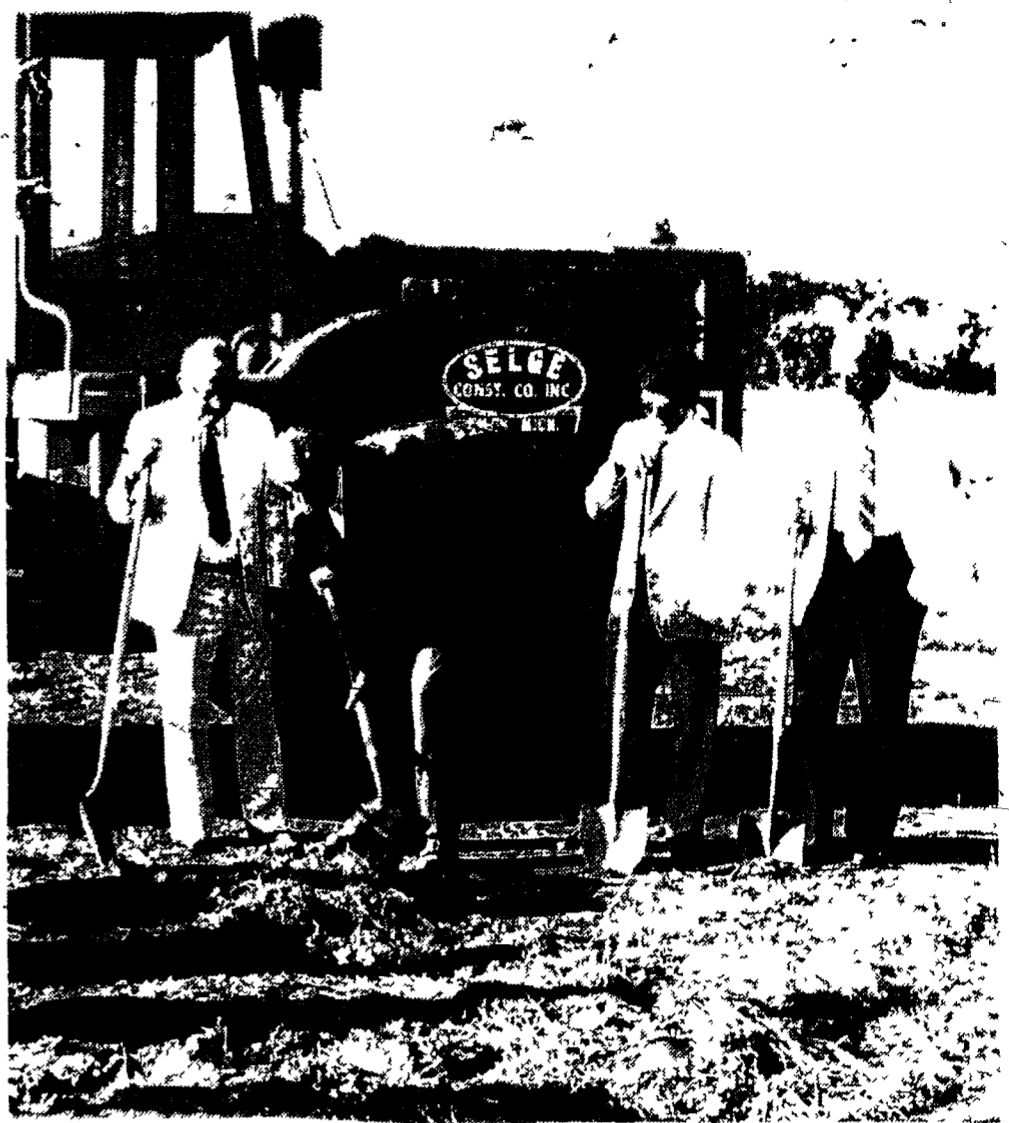
The groundbreaking ceremony for the water and sewer project for Andrews Farm Industrial Park was held in June. Above, Harry Kennedy, left, president of McCoy Creek Development Corp., watches as Mayor Ray Berry tosses the first shovel-load of dirt at the site. Also watching are Tom Deneau, engineer, and Clyde Remmo, city manager. (BCR file photos)
