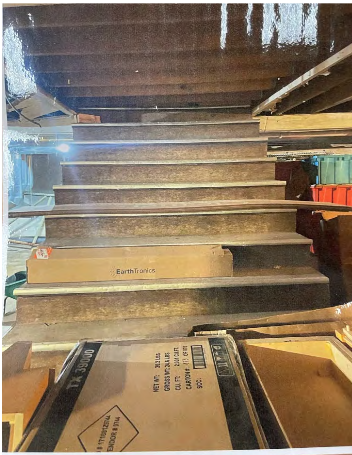
The steps that go into the basement of the store under the Front Street entrance. Photo provided by Joe Krueger
