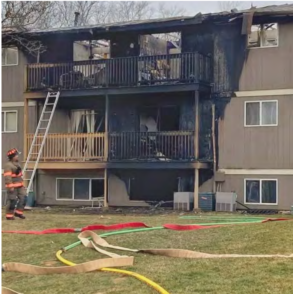
Fire destruction of Building G, March 15 2021, Photo by Nik Sanchez
