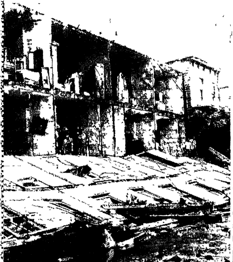
TORNADO DAMAGE . . . Amazed home-dwellers find themselves with plenty of air conditioning as a result of a 90-mile-an-hour tornado that ripped through Richmond, Virginia. At least 50 persons were injured, hundreds were left homeless, and property damage was estimated in the millions. House above was in 25-block-section-ripped-by-the-tornado. The entire front wall of the two-story structure was neatly ripped off, producing house with a view.
