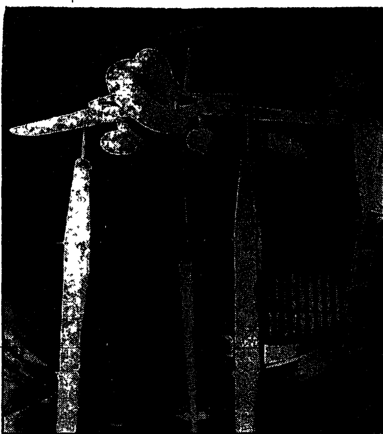
STILL FLIGHT —Mounted in the 19-foot pressure tunnel at Langley Aeronautical Laboratory, Langley Field, Va., a scale-model plane is about to be tested for stability and control. The tunnel will be filled with a rushing torrent of air speeding at 200 miles per hour. Pressure will increase two and one-third times.
